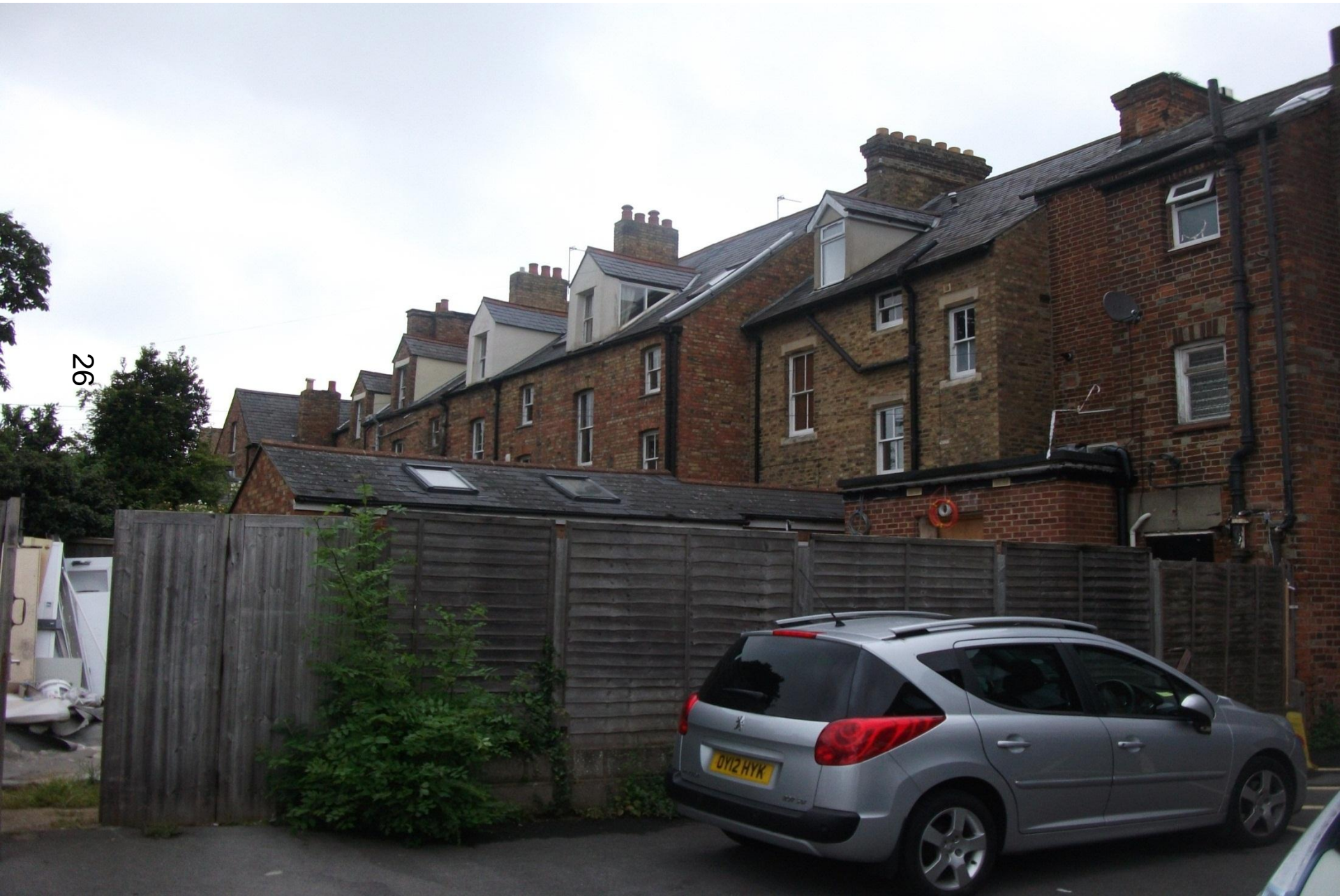
View of the Rear of the Wider Terrace of Houses from Health Centre Parking Court
